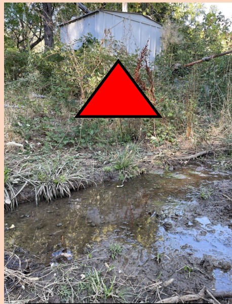
Natural springs pushing up
