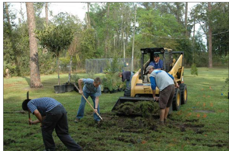
FIGURE 8.2: After cutting the sod into strips, patches can be lifted by hand or using shovels.
