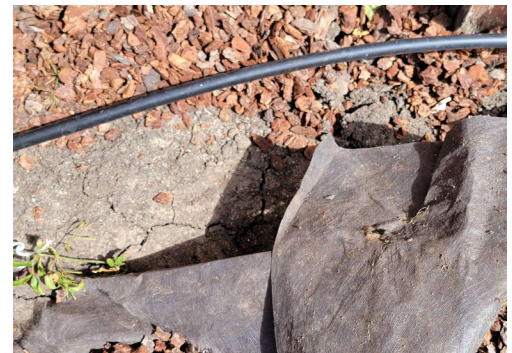
Dry cracked soil beneath fabric
